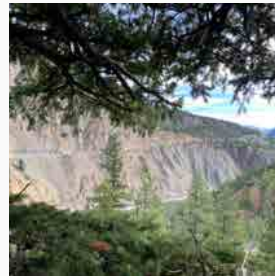
BIG SLIDE ON HWY 12 FROM THE TEXAS CREEK SIDE
